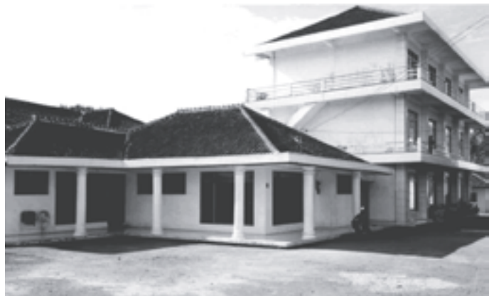
Main buildings at a pesantrén . The residential area of the Kiai to the left, male dormitories to the right. Photo J. Hellman
